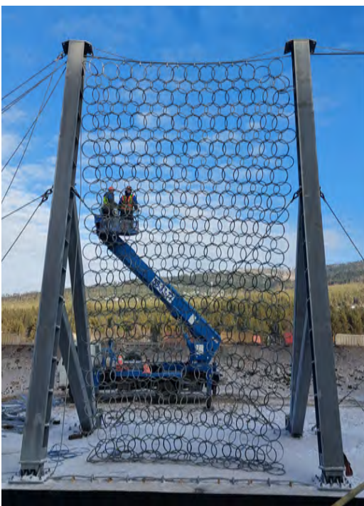
Ring net 4.42.19/6 for debris flow barrier
