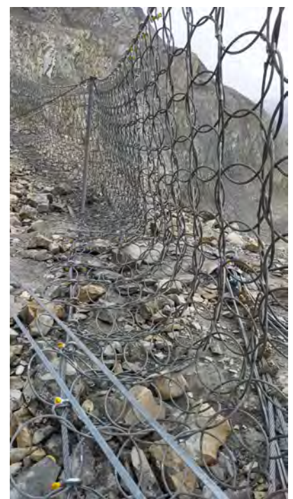
Ring net 3.25.7/6 for rockfall barrier
